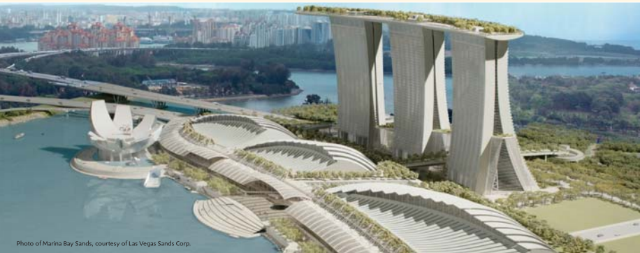
Photo of Marina Bay Sands, courtesy of Las Vegas Sands Corp.
